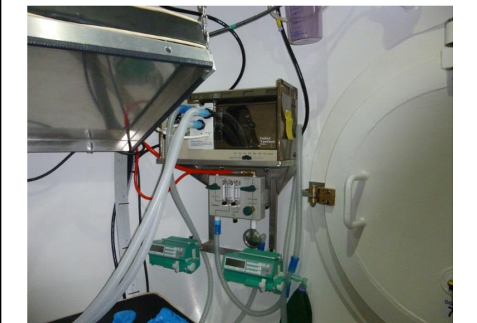
A penlon ventilator and hyperbaric syringe pumps. Inside the BP Baku HRF
