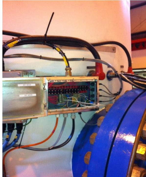
Figure 7. AED External chamber connections
